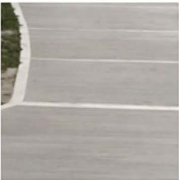
Brushed Concrete with trowel edge finish (streets)
